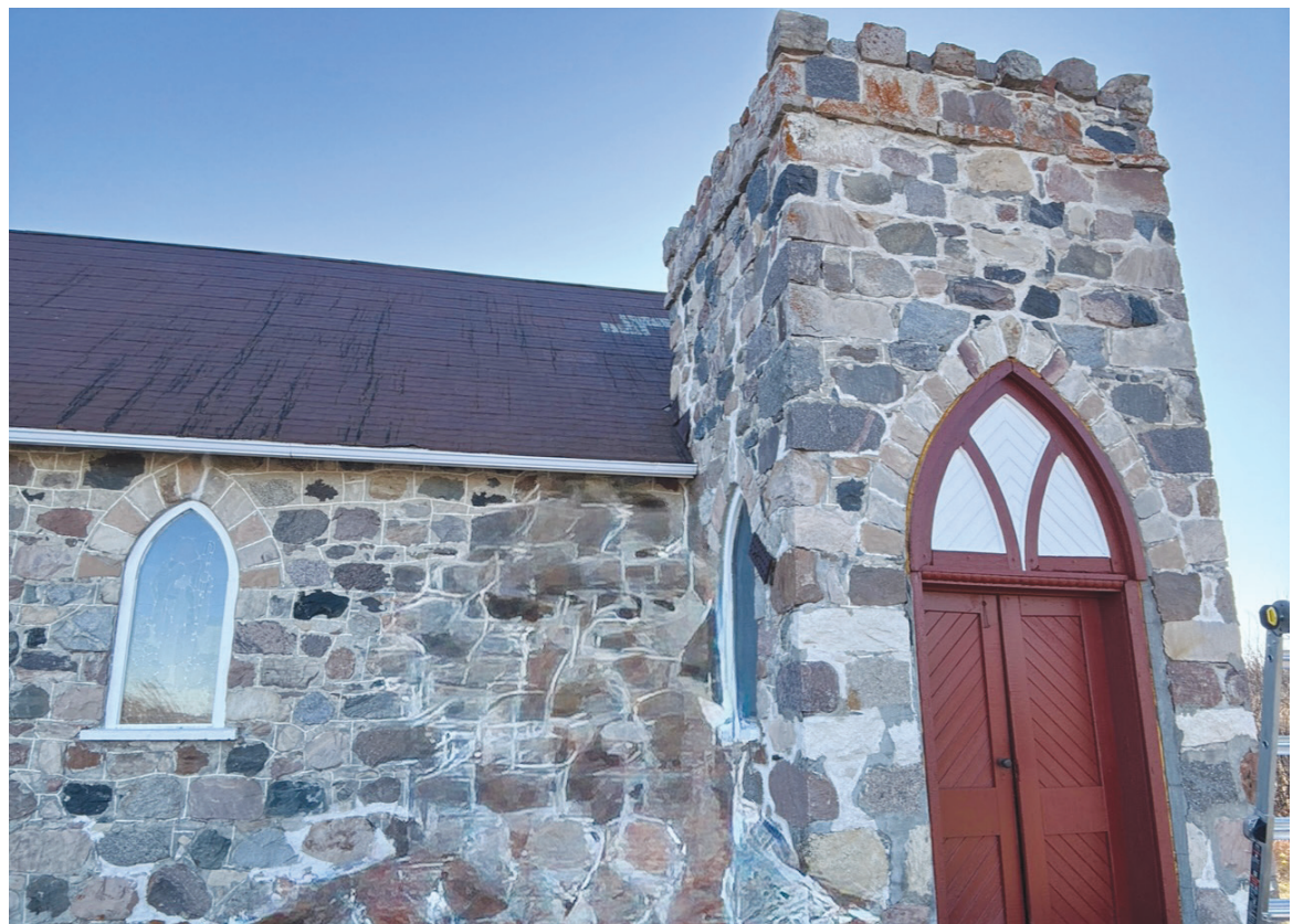
When St. Thomas' Church, Vernon, located midway between McLean and Qu'Appelle was constructed in 1898-99 no one realized that the flat roof in the tower would be prone to developing minor leaks over the years. But leak it did, and various repairs have been done over the years. Photos by Bruce Farrer
